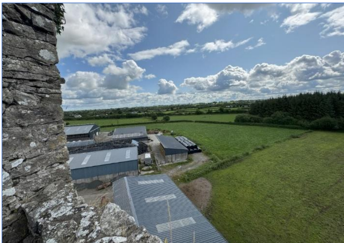
Figure 4: Parapet view ENE towards Brittas, c.4.5km distant. View constrained by doorway access from spiral stair on left (LDARCH 2025).
